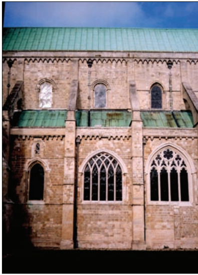
Exterior of South Quire Aisle
