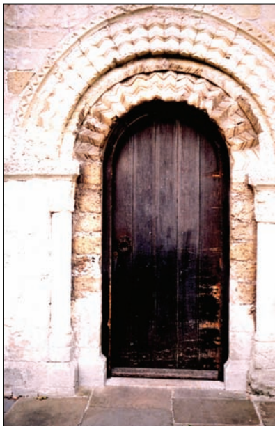
12th-century doorway on south side of Southwest Tower
