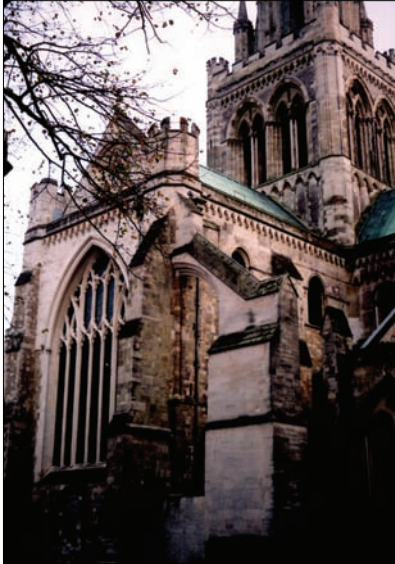
North Transept and Buttriss 60
