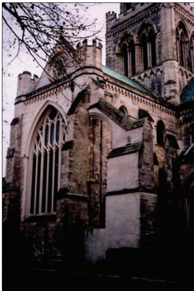
North Transept with Buttress 60
