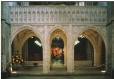
The Arundel Screen after re-instatement, 1960
