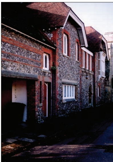
The street front onto Canon Lane
