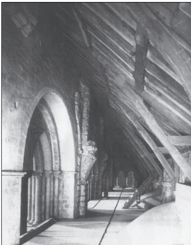
The medieval roof above the North Aisle
