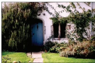
Surviving doorway and window of one of the early 15th-century houses in Vicars' Close
