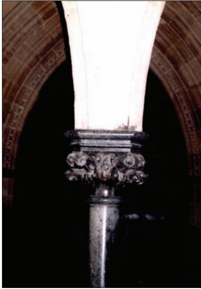
Purbeck marble capital to the slender central shaft at the entrance to St Richard's Porch
