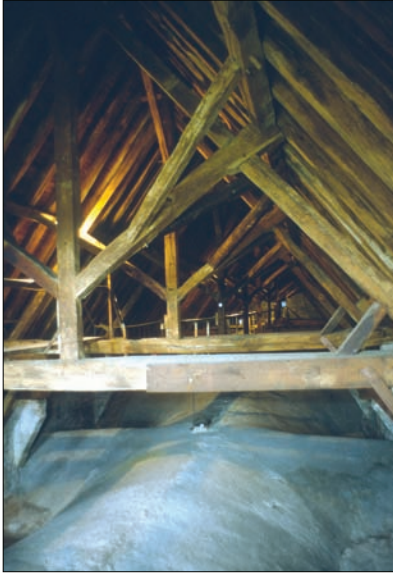
Above the vault, the late 13th-century roof of the Nave, looking east before fire compartmentation in the 1990s
